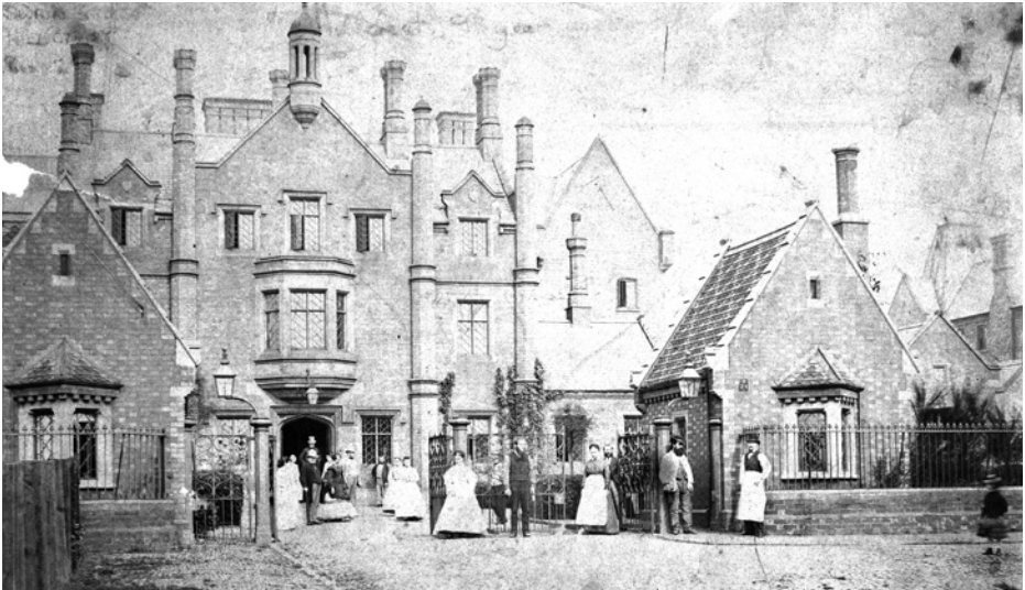
Hillcrest Workhouse, 'Union House' 1890, the record office for Leicestershire, Leicester and Rutland
